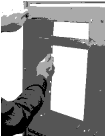
Insert the left reinforcement plate into the mounting cut-out.
